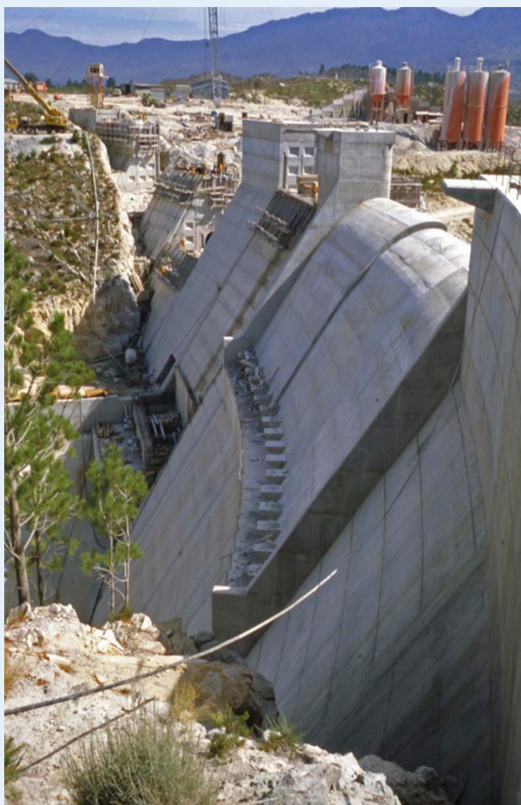
Kogelberg Dam nearing completion as part of the Palmiet Pumped Storage Scheme. The dam features a two-level spillway that is a 45 m-long uncontrolled crest in the river section.
